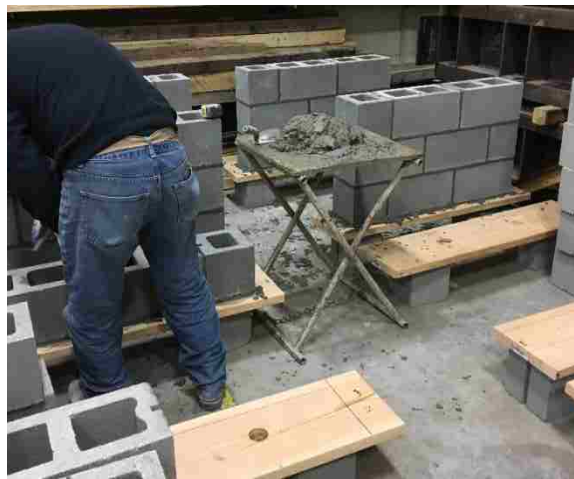
Figure 3-4: Masonry Panel Construction
